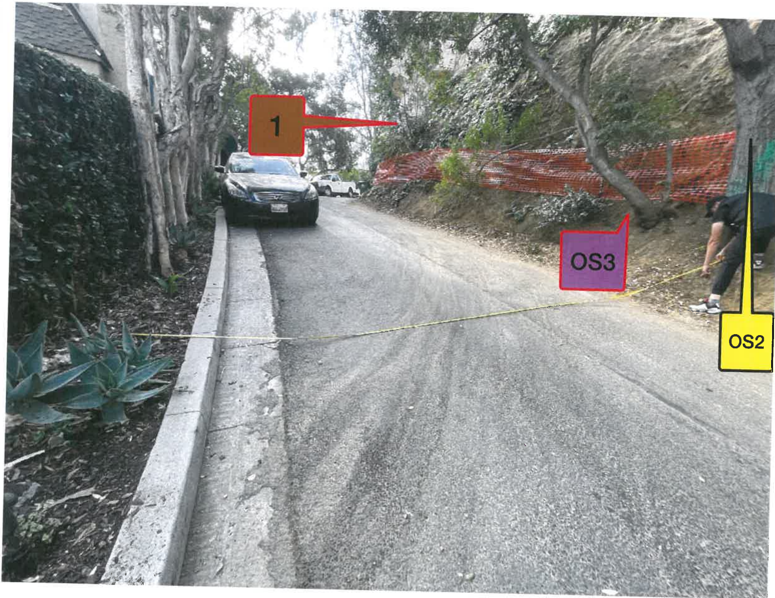
PHOTO 11 - Shows front slope and steep terrain. House will be built directly into hillside. The small Toyon shrub #1 is located directly on the steepest portion of the front slope. This photo is also showing the back of curb location of the required widening of the road.
